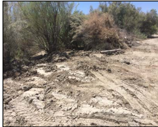
Post-project inspection, October 2017
