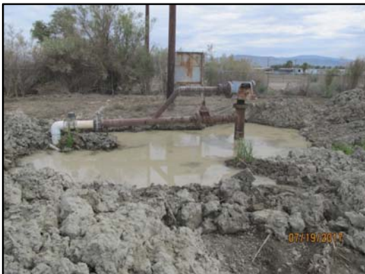
Pre-project inspection, July 2017
