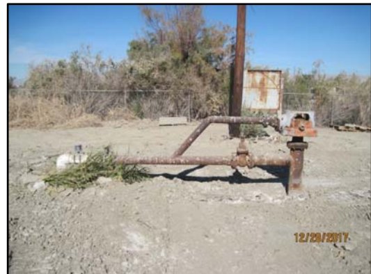
Post-project inspection, December 2017
