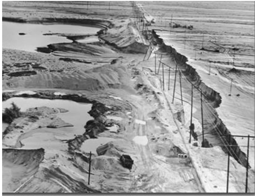
Figure 3-4: Whitewater River at Indian Avenue as it appeared on March 23, 1965. Indian Avenue was destroyed by flood waters cutting back from a sand and gravel pit on the downstream side.
