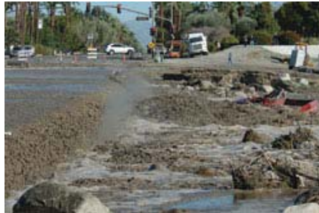
Flash Flooding Results in Property Damage
