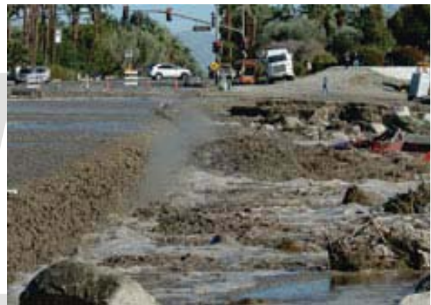
CVWD's Stormwater Facilities Provide Flood Protection
