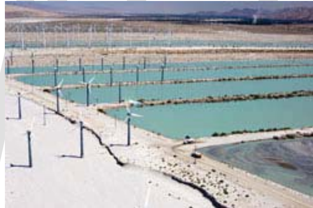
Whitewater Spreading Area at Windy Point
