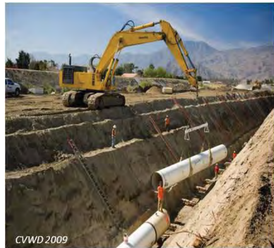
Installation of 54-inch Mid-Valley Pipeline for Delivering Recycled Water
