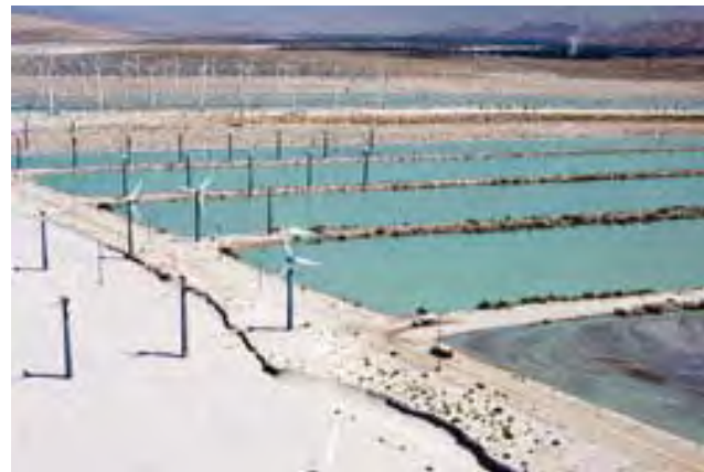
Whitewater Spreading Area at Windy Point
