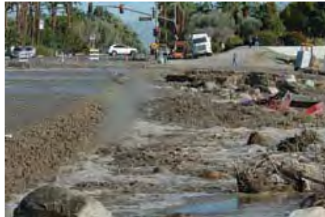
Flash Flooding Results in Property Damage
