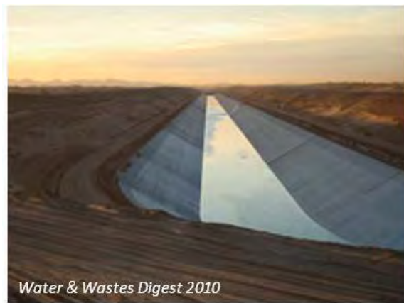
Coachella Canal Lining Project
