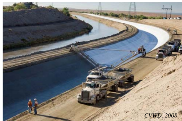
Coachella Canal lining project
