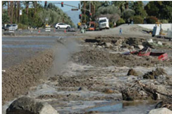
Flash Flooding Results in Property Damage
