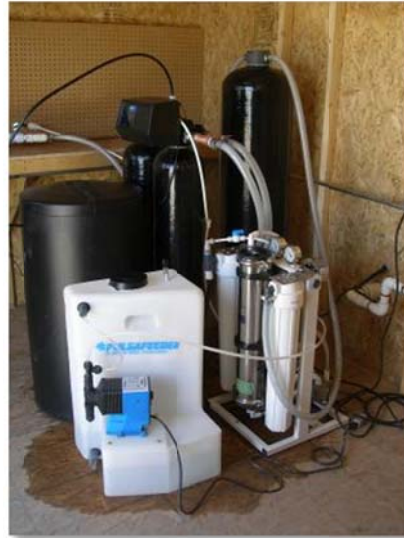
Reverse Osmosis System used to remove arsenic from drinking water Credit: Sergio Carranza, Pueblo Unido Community Development Corporation
