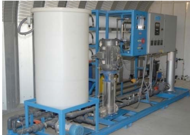
Agricultural Drain Water Desalination Pilot Facility Source: 2010 Coachella Valley WMP
