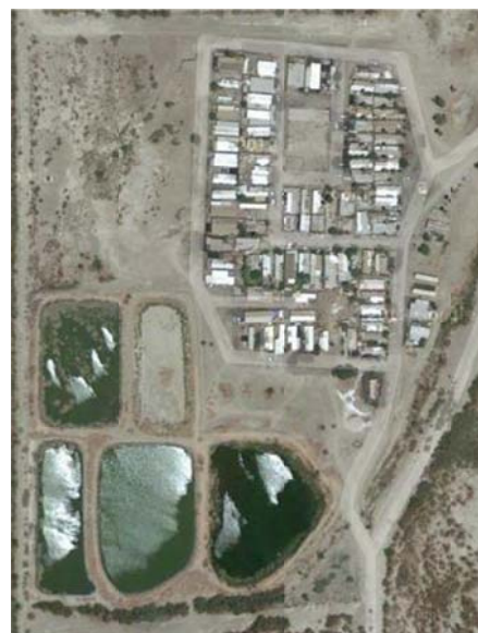
Existing Wastewater Lagoons in the East Valley (Mecca)
